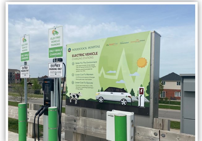
As well as 21 electric car charging stations, educational signage has been installed to promote the importance of reducing CO2 emissions.
