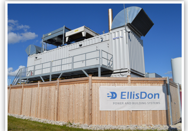
The hospital's Combined Heat and Power Cogeneration Plant provides heat for WH and produces 85% of its electricity needs.
