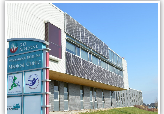
Along with the 340 roof-mounted solar panels, these facade-mounted panels produce 50% of the power for the WH Medical Clinic.
