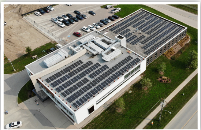
Aerial photo of solar panels on the Medical Professional Building off of Athlone Avenue.
